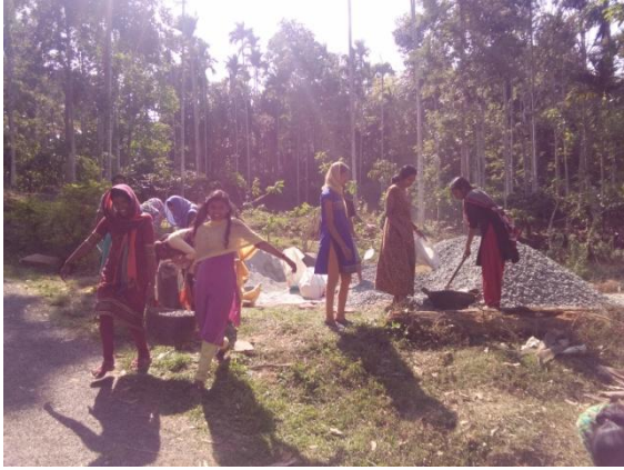
Supporting house construction
